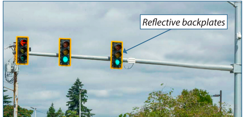
Above: Safety improvements include installing reflective backplates for traffic signal heads.
